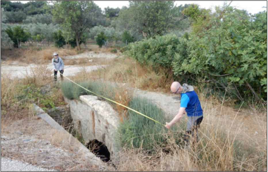
HSS/079 – ‘Stone Bridge’ from the north east in September 2024. Marks on the bridge elevation are due to plant growth. The olive grove in the background was the site of the local Ottoman commander’s headquarters on 25 April 1915. Photos this page see pages 52 - 57.
