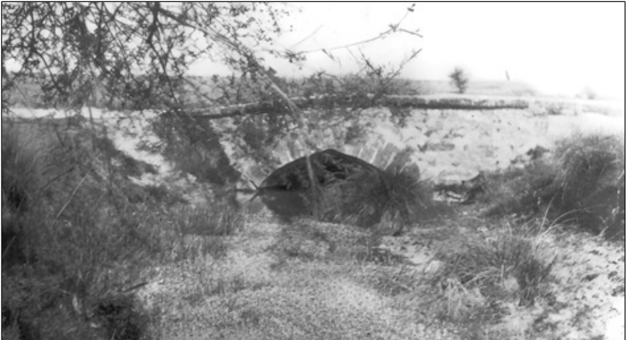
HSS/079 - 'Stone Bridge,' from the south east, taken either during the campaign or in the post-war occupation period. See modern day photo of 'Stone Bridge' in the colour section.
