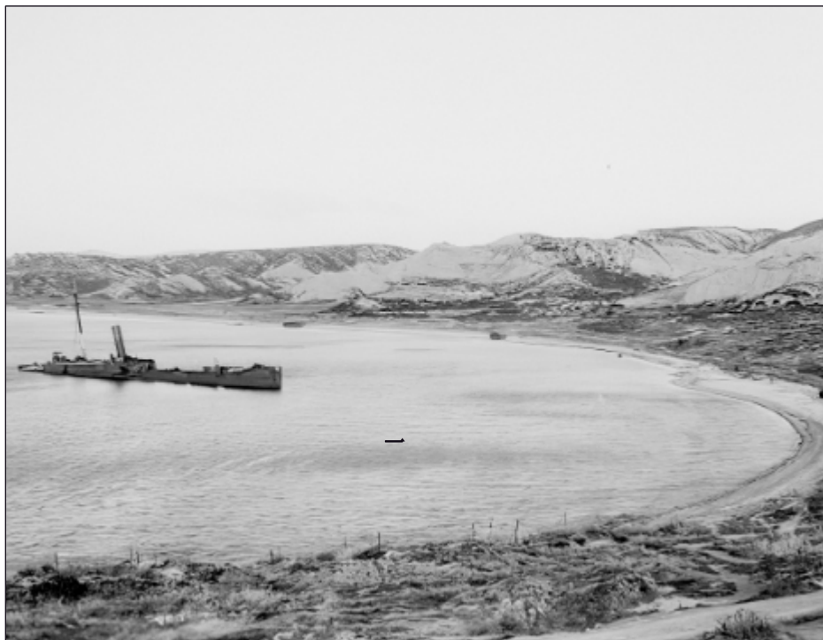
The British Director of Works steamer, Milo , was sunk off North Beach and filled with sand on 26 October 1915 to act as a breakwater for Walker's and William's Piers. See colour photo page 32.
