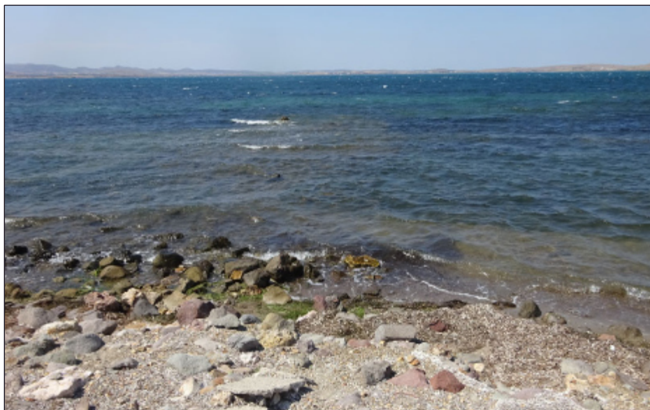
Broken sections of a concrete skim indicate the landward platform of the pier. Waves can be seen breaking over the submerged remains. This photo and above right by Nick Baker. See pp 5-8.
