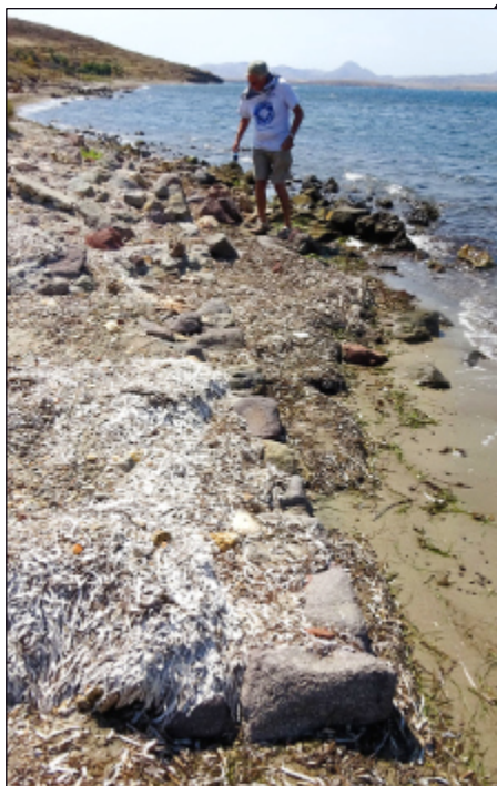
A straight edge of boulders set in concrete mark the landward edge of Sports Pier, Lemnos.
