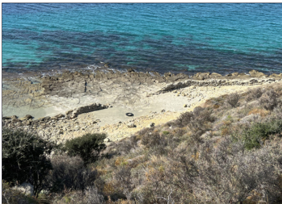
The well-preserved section of the coast road retaining wall at the western end of Tekke Burnu.
