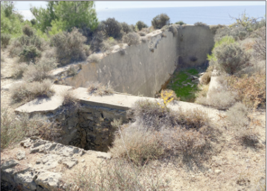
Water Tank HSS/016A on Hill 114 taken from the north east.
