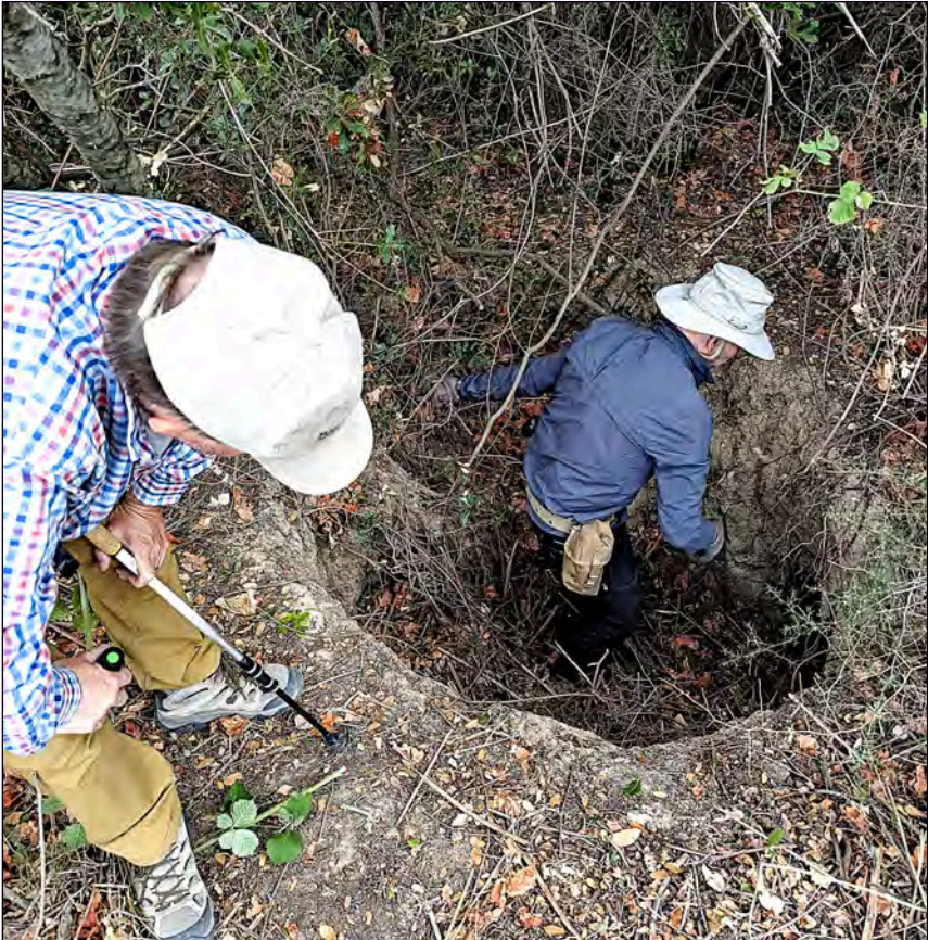
HSS/o62 – Collapsed dug-out in No.1 Australian Line. See Map 2 page 36.
