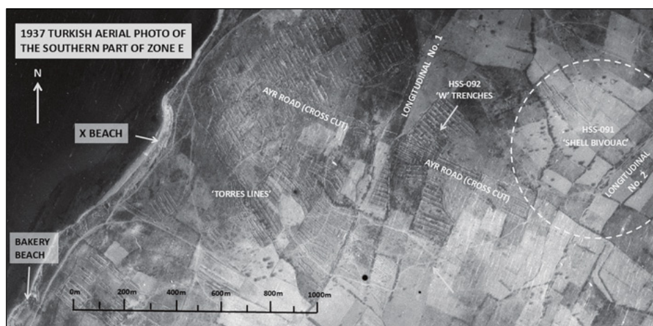
Fig. 2: HSS-091 & HSS-092 shown on a 1937 Turkish aerial photograph. The outlines of the many ‘W’ section bivouac trenches which covered the area in the second half of the campaign can be clearly seen. The tree lined field boundary running through the western part of ‘Shell Bivouac’ still exists today – see Site Map No. 1, in the colour section of this edition (page 30).
