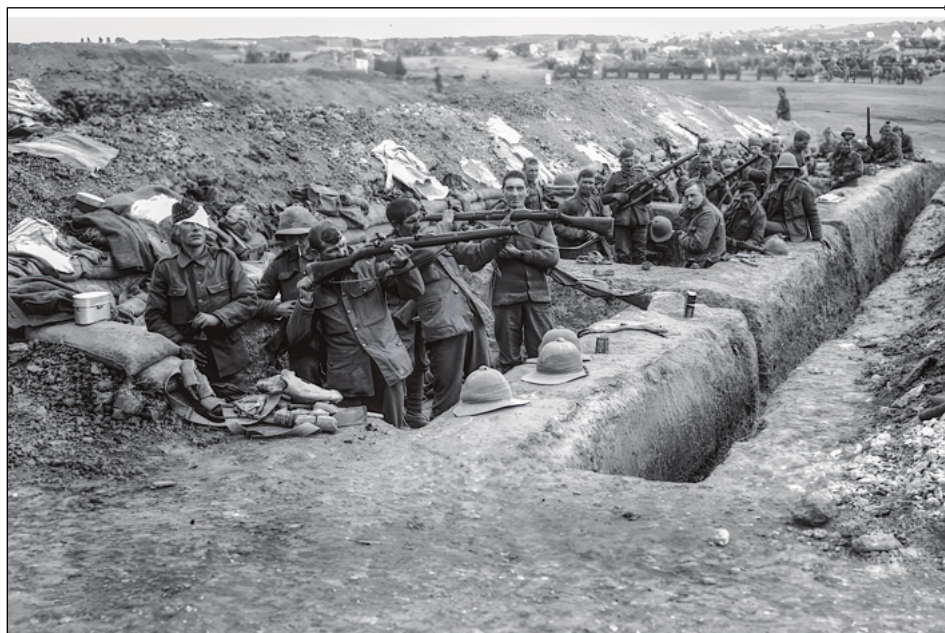
Fig. 5: Troops of the 52nd Division at Helles. The trench follows the standard pattern of two parallel trenches, divided by a flat section, with protective banks on either flank. Later versions were lined and traversed with sandbags. The southern end of Gully Spur can be seen in the distance on the right, placing the trench in a similar position to those at HSS-092.
