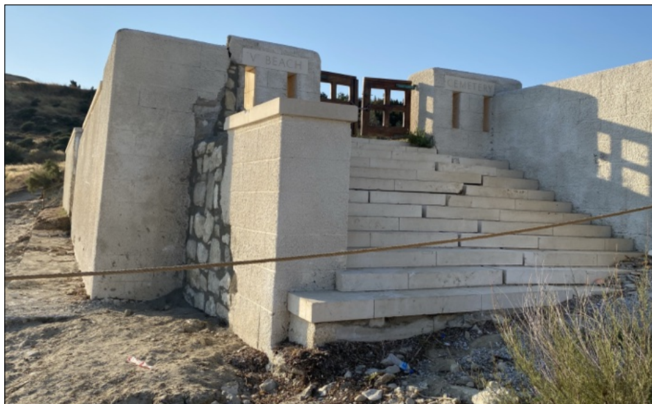
Storm damage to V Beach Cemetery, Helles, seaward entrance, 11 August 2026. Photo courtesy Serpil and Bill Sellars. See page 66.
