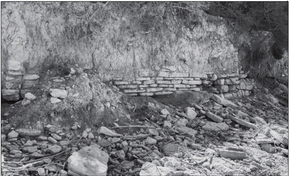
Fig. 8: HSS-098 – The retaining wall of a lean-to shelter at Gully Beach, situated 100 metres north of the mouth of Gully Ravine.
