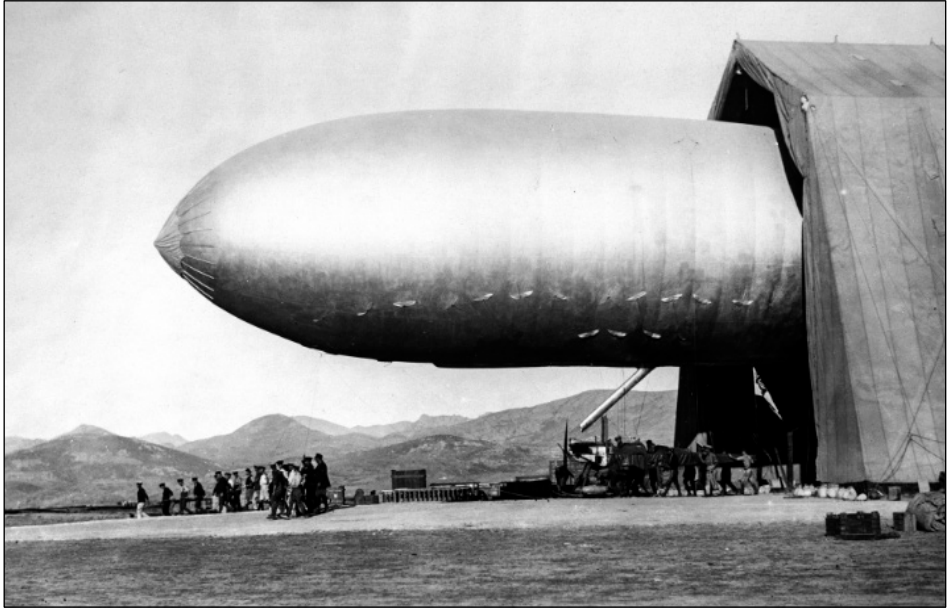
The airship being walked out of the southern door of its shed, with a view to the high ground across Kephalos Bay. The picture is a beautifully composed photograph, probably taken by Ernest Brooks, but its purpose was utilitarian. Flight Commander Sparling wanted to illustrate to the Admiralty 'how close the car must be kept to the ground to prevent envelope touching the shed.'
