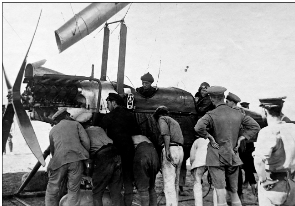
A good view of the car, a modified B.E.2 aeroplane fuselage with its wheeled undercarriage replaced by skids and floats. Note the blower tube in the slipstream of the propeller, which allowed the crew to force air into the ballonets.
