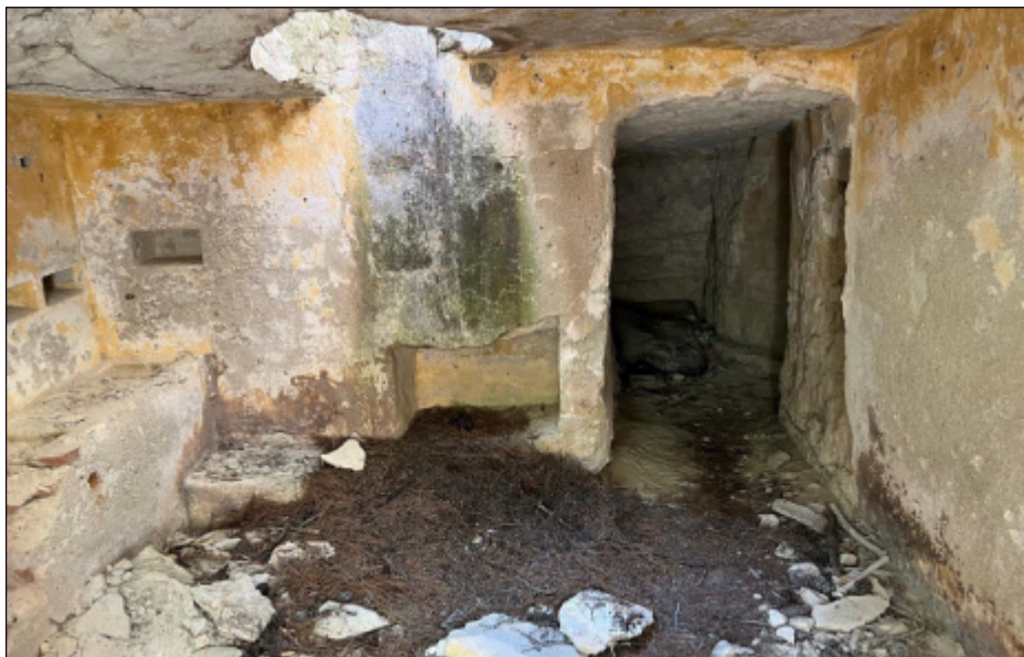
HSS/o04/DO/o2 - Main room in the 'Command Post dug-out' showing the corridor & annexe. Entrance to the 2nd room on the right.
