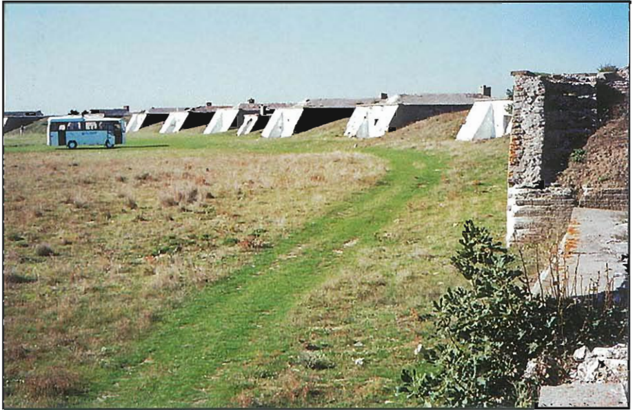
Fort Sultan – The Lines of Bulair, October 2006
