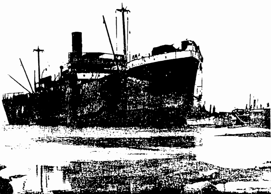
SS 'RIVER CLYDE' AT V BEACH 25 APRIL 1915
