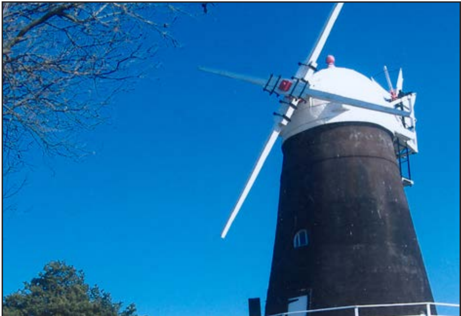
Barnham Mill, the home of SQMS Percy J Baker [Pages 18–19] Photograph by Frances Stanley
