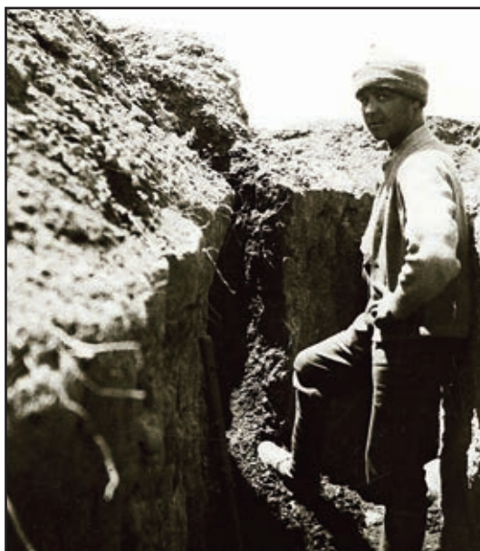
Digging a Sap
