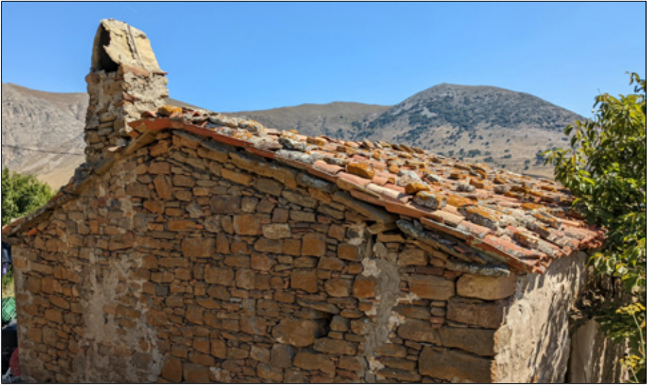
Figure 6. A Greek two-storey building in Kaleköy that shows their typical construction. See pages 48 - 58.
