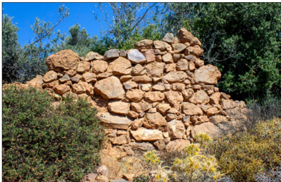
Figure 5. Remaining courses of the stone wall at the top of Eşelek village.
